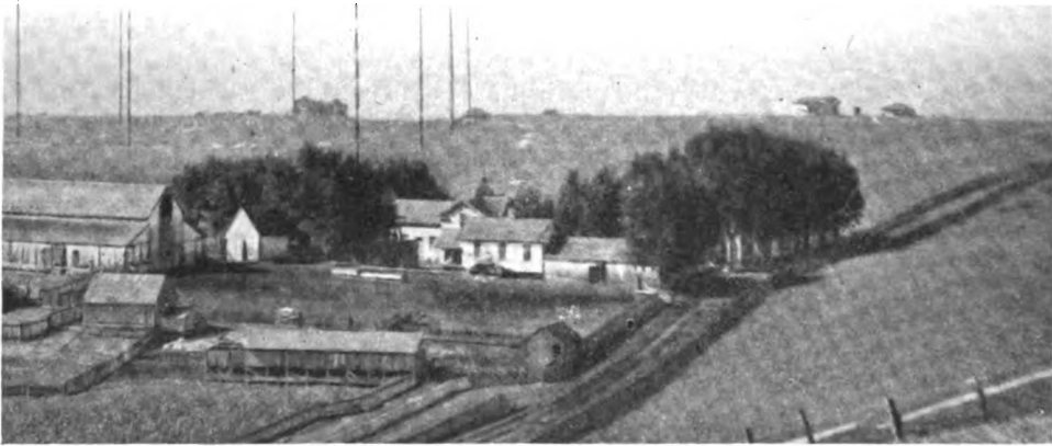
A rear view of the mast line of Bolinas, the transmitting station of the Marconi trans-Pacific wireless link in California, from the ranch buildings, in the foreground, adjacent to the station property. The line of masts is a mile in length, extending to the ocean. In the background are shown the power house and the Marconi hotel for engineers and operators. Messages destined for Hawaii and Japan are flashed from this station
