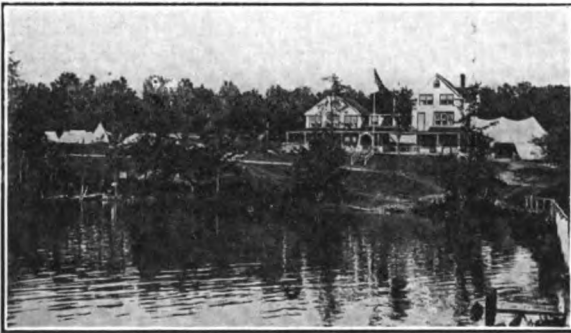
The double-page photograph across the top shows the company streets from the senior end, also the 250-foot aerial, suspended from trees. The center photograph gives a view of Birchwood Lake, the club house and mess tent showing in right of background
