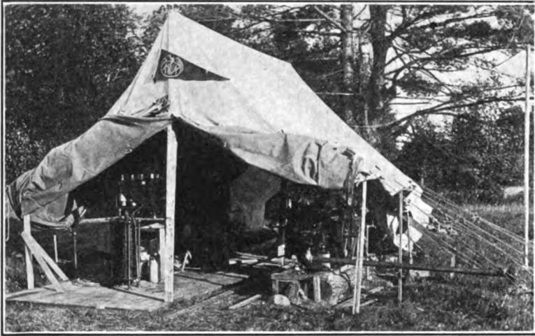
Above, the military headquarters' wireless station, giving a glimpse of the condenser rack and the 8 h. p. Lawbanks-Morse engine used for generating power for the 2 k.w. set loaned by the Marconi Company. Both engine and wireless apparatus were donated by the respective makers in the interests of patriotism. In center, Officer of the Day on inspection rounds
