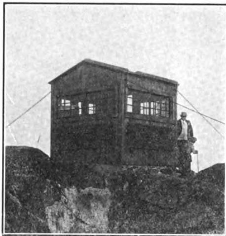
The forest-fire warden's house which provided protection for the author of this article and his companion during a storm
